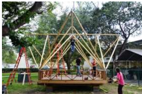
Fig. 3. Testing the framing of the Everglades Eco Tent project, University of Miami Design/Build, 2012 (photograph by Jim Adamson)
