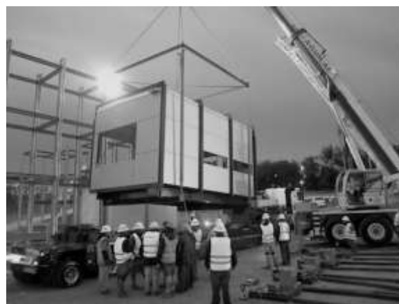
Fig. 4. Lifting and placing the living room module (photograph by Clay Anderson)
