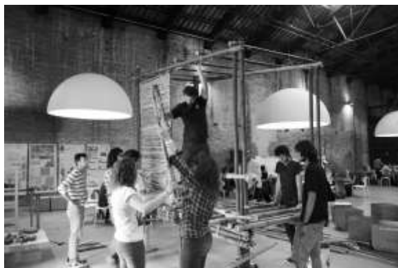
Fig. 4. TLT stage 4: building the bamboo prototype
